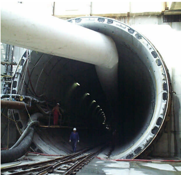
Application in tunnelling
